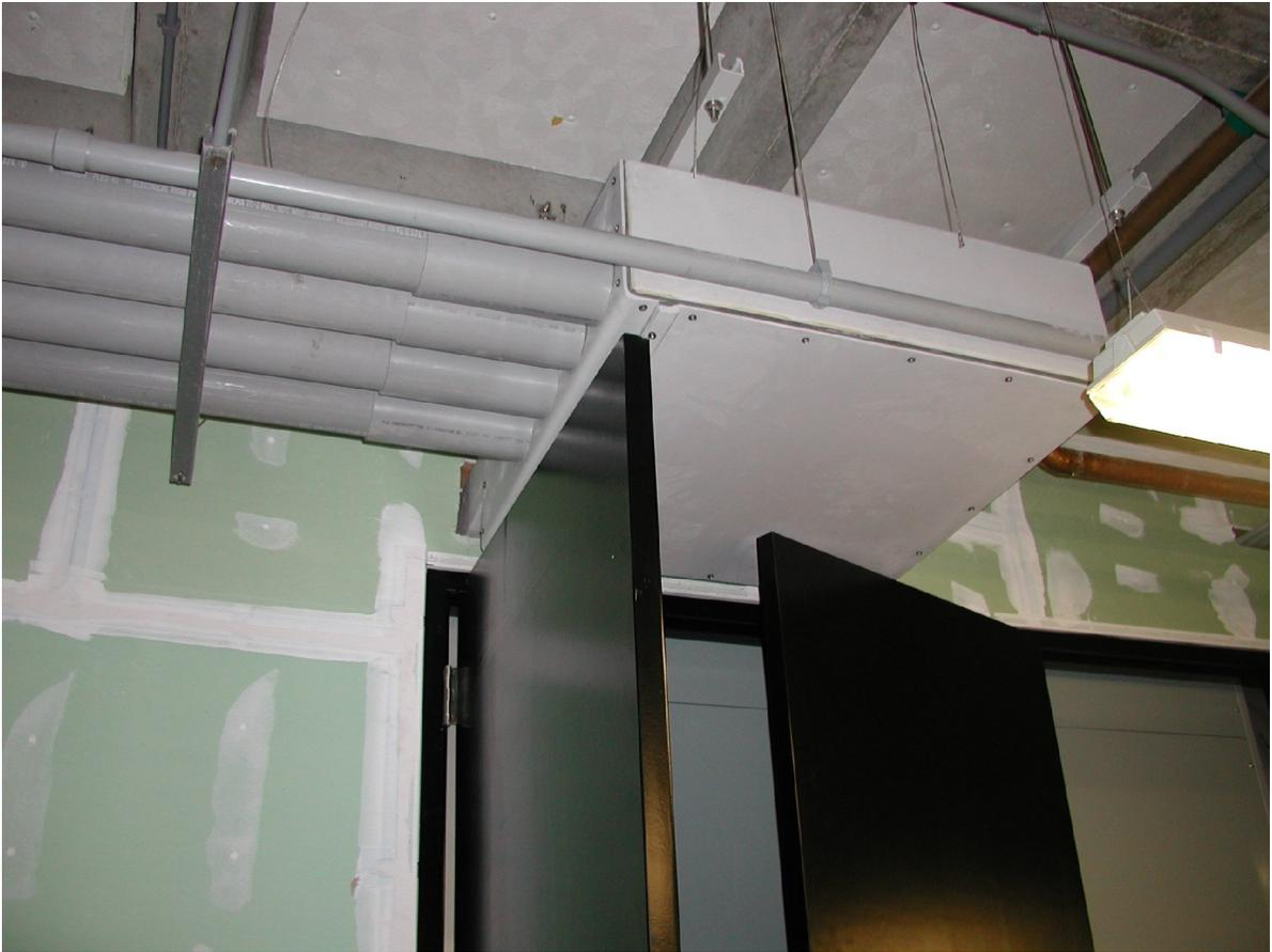
**The Results: A properly customized enclosure that handles the corrosive environment in the Monterey Bay Aquarium wash down room**
